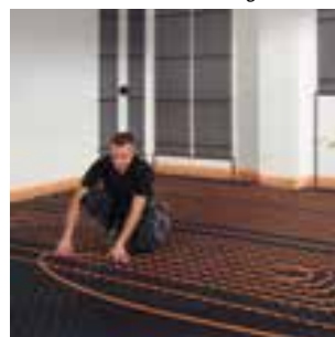
Underfloor heating living area
